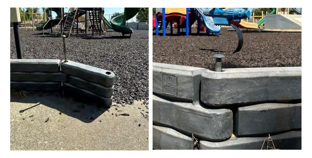
If some of the **pins** that hold the barriers in place are missing or sticking out of place, they should be fixed or replaced. Ensuring that the pins are securely in place will help maintain the integrity of the barriers and prevent any potential hazards.
