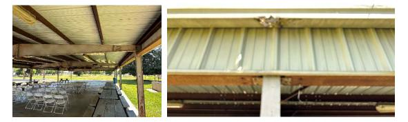
Attend to the **gutter** repair needs of the pavilion to prevent water damage and ensure proper drainage during rain. Repair any leaks or damages to the gutters to maintain the structural integrity of the pavilion.
