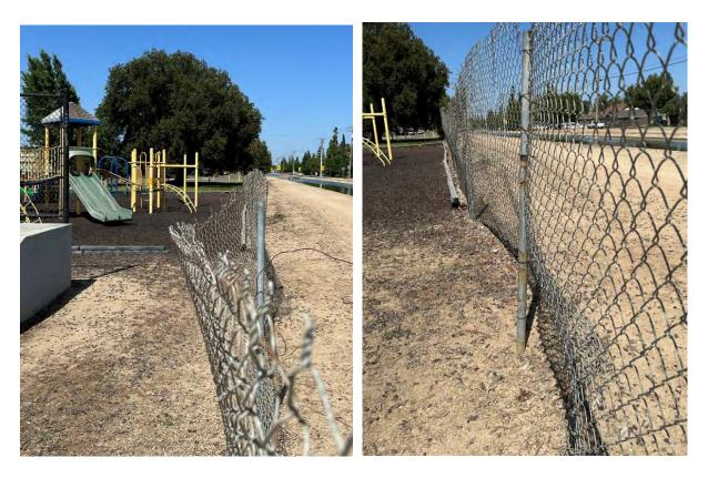
Repairing the falling **fence** along the park and canal is crucial for both safety and aesthetics. Inspect the fence thoroughly and identify sections that require immediate repair or replacement. Missing fence posts should be replaced to ensure the overall integrity of the fence.
