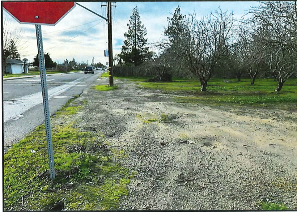
East edge of the site, looking south along North Reinway Avenue from the northeast corner of the site; 01/12/23.
